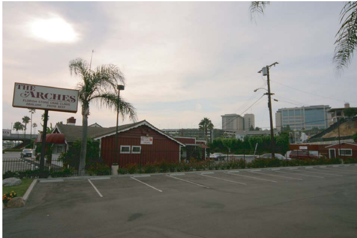
View 15: View from the South side of Arches on West Coast Highway.
