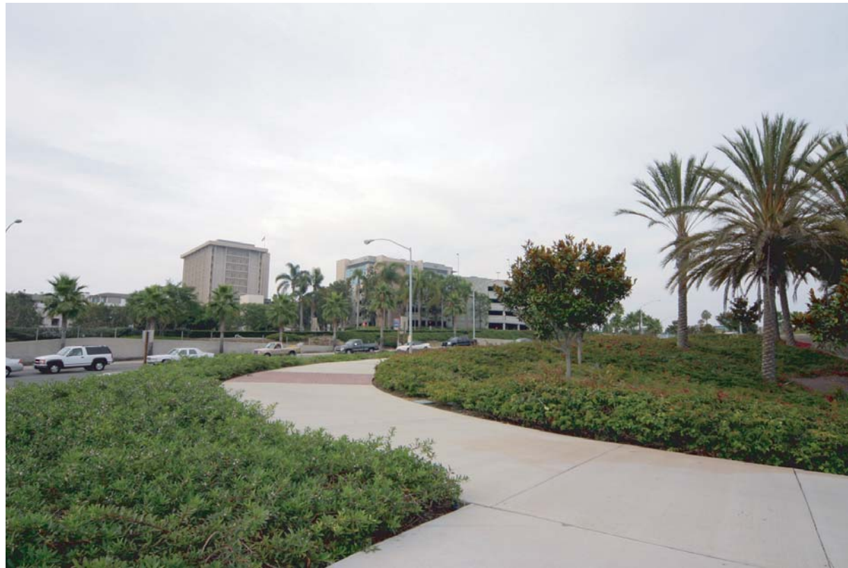
View 17: View from West Coast Highway.
