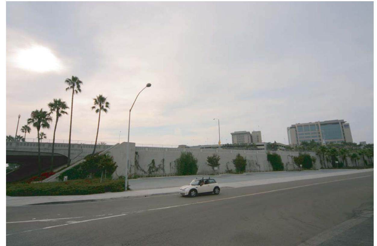
View 16: View from Old Newport Avenue.
